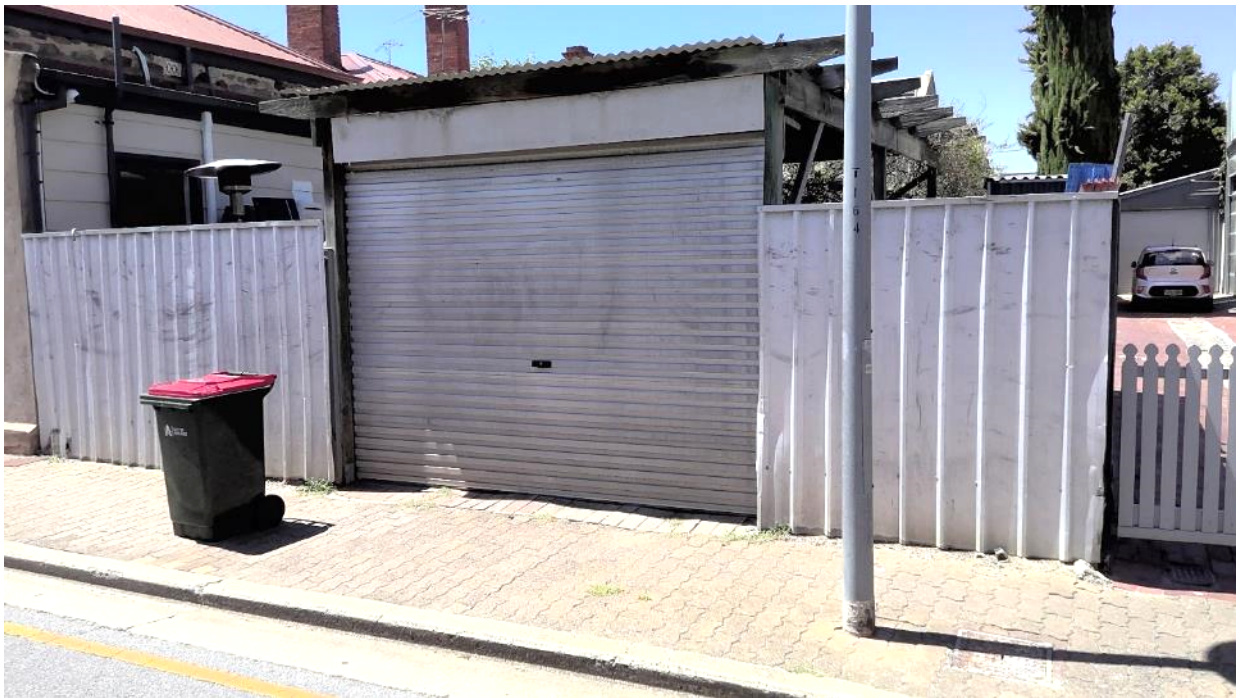
Photo 3.2 – View of roller door on Corryton Street frontage
